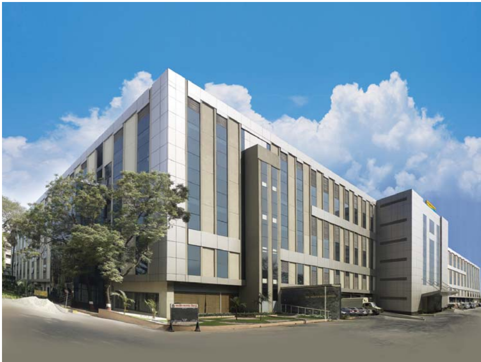
Switchgear Factory, Mumbai
